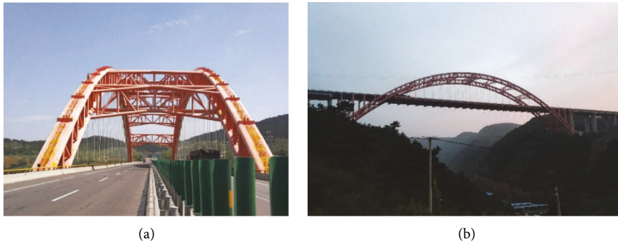
FIGURE 1: Beisheng CFST arch bridge. (a) Arch bridge lane. (b) Overall state of an arch bridge.
