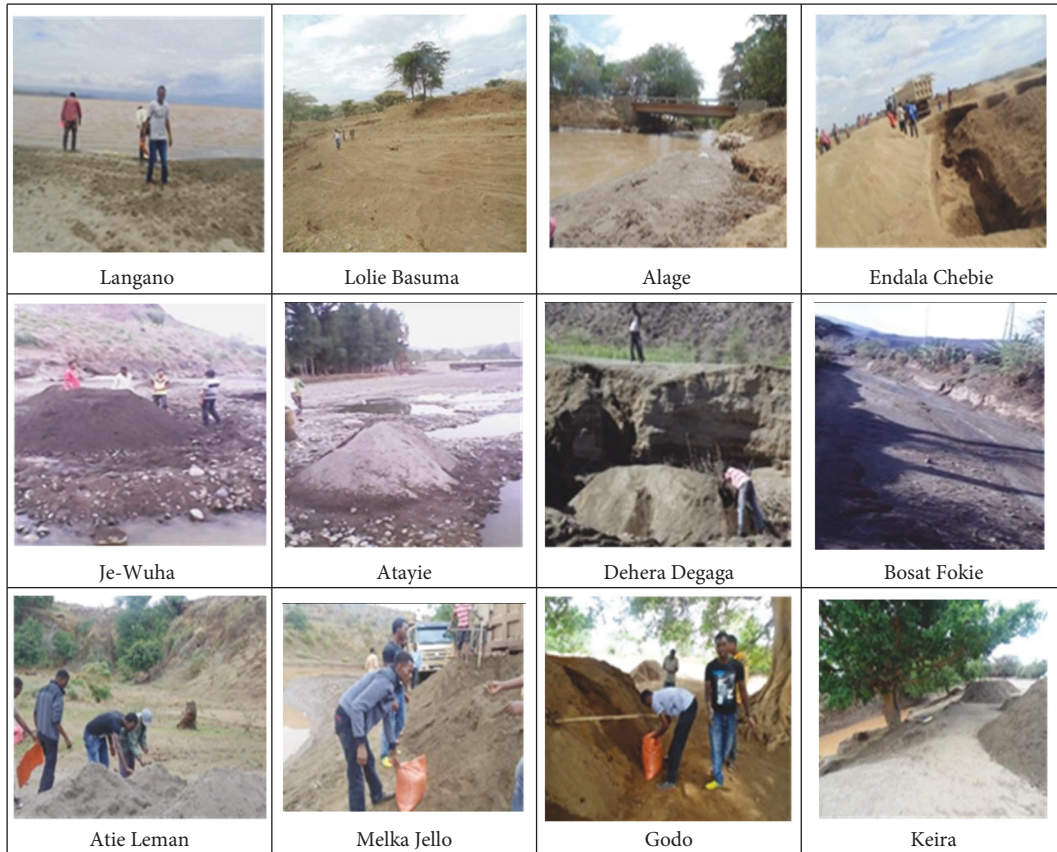
FIGURE 1: Quarry sites captured overview (source: captured during sample collection from source).
