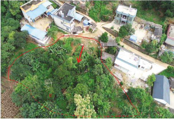
FIGURE 15: Aerial view of the Dawanjiang landslide.
