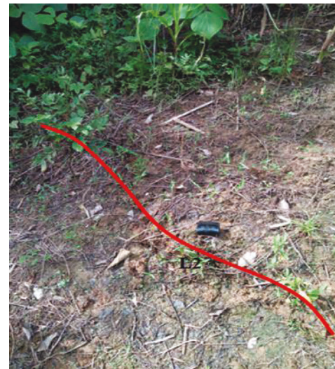
FIGURE 17: Leading edge bulging of the landslide.
