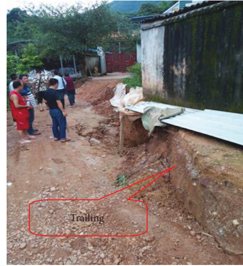
FIGURE 16: Trailing edge boundary of the landslide.
