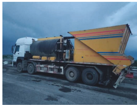
FIGURE 17: Spreading process of synchronous gravel seal car.
