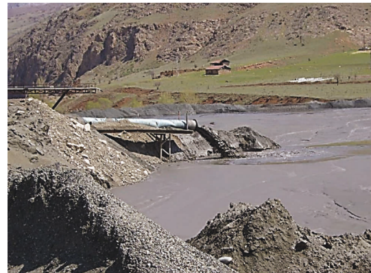
FIGURE 2: Discharge of iron ore processing waste into the waste pond.
