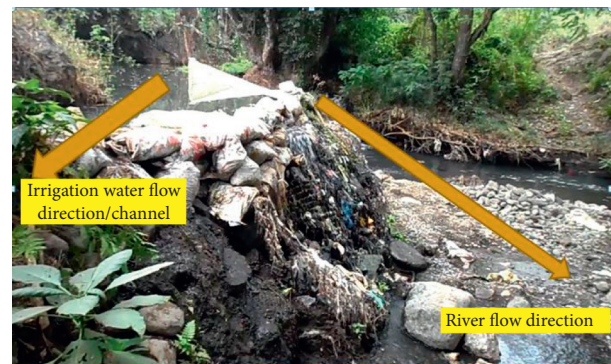
FIGURE 5: Furrow intake constructed with sand bag/stone/trees logs.
