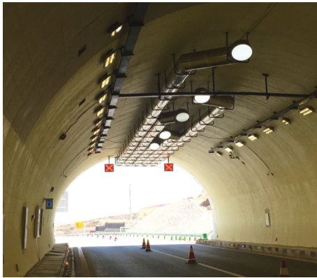
FIGURE 8: Light pipe installation in plan zone of Huashuyan Tunnel.
