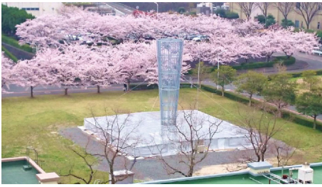
FIGURE 15: The wind solar tower prototype in Chikushi Campus, Kyushu University.
