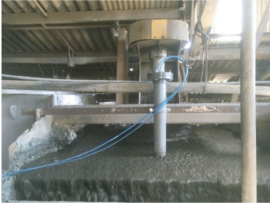
FIGURE 12: Sensor installation at Minera Don Alberto site.
