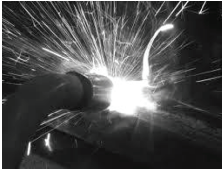
FIGURE 2: Opening for electric arc welding activity.
